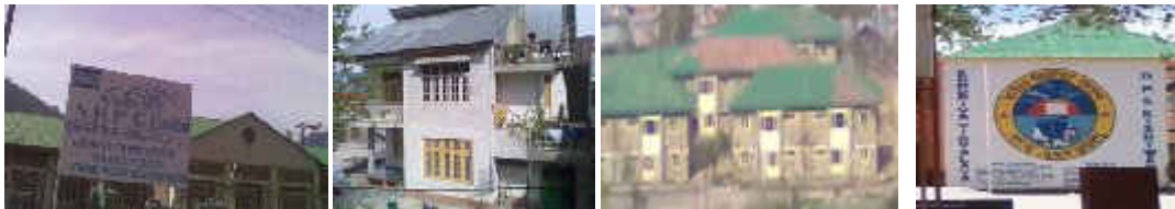
Above Photographs reflect a new scenario of district kishtwar after the construction of DHP Power Project from left photograph 1. Power Grid Station NHPC kishtwar. 2. Pacca House after getting compensation. 3. NHPC colony in semena area. 4. KV school for all children's opened by NHPC.
